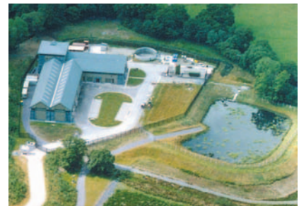
Example of remote pumping station.
